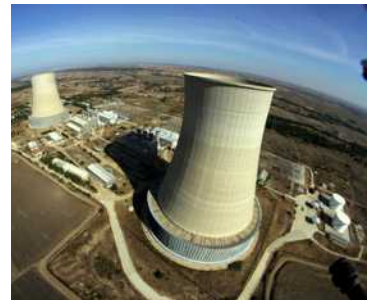
Power Plant Chargers
